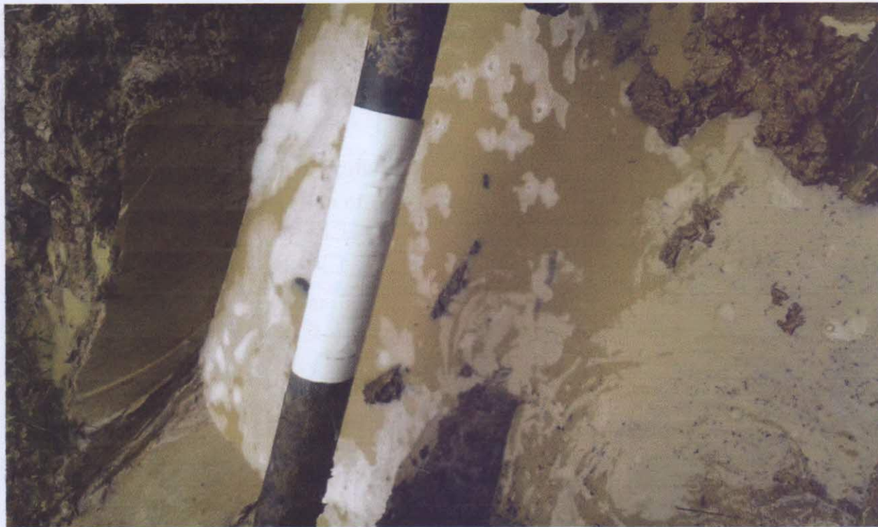
LEAK POINT REPAIRED AND WRAPPED
